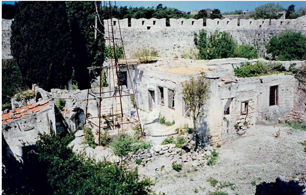
FIGURE 1: The site in early 1996 after a first cleaning
