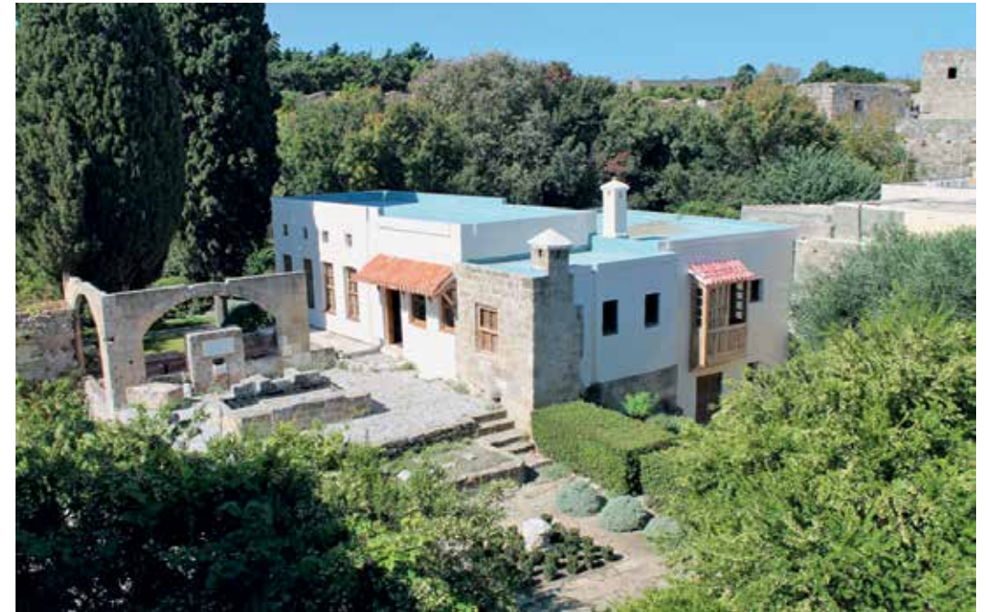
FIGURE 2: The site in April 2000 after the completion of the restoration
