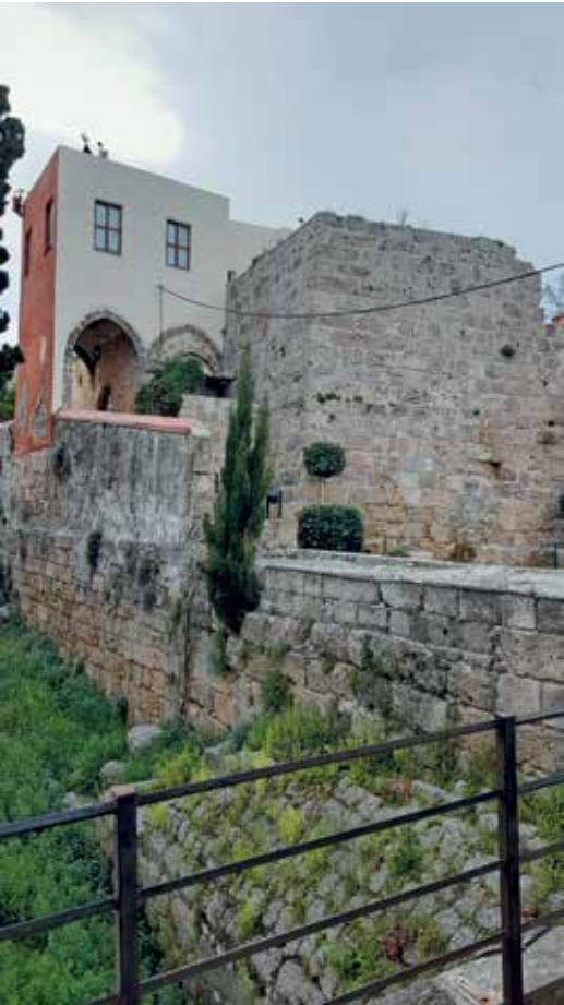
FIGURE 8: Ahmed Fethi Pasha's Old School, Rüştiye above Byzantine and Medieval walls Photo: G. Ntellas, 2025
