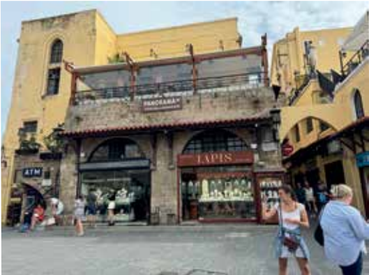
FIGURE 9: View of the medieval ground-floor building with the cross-vaults (Loggia) in its current form.
